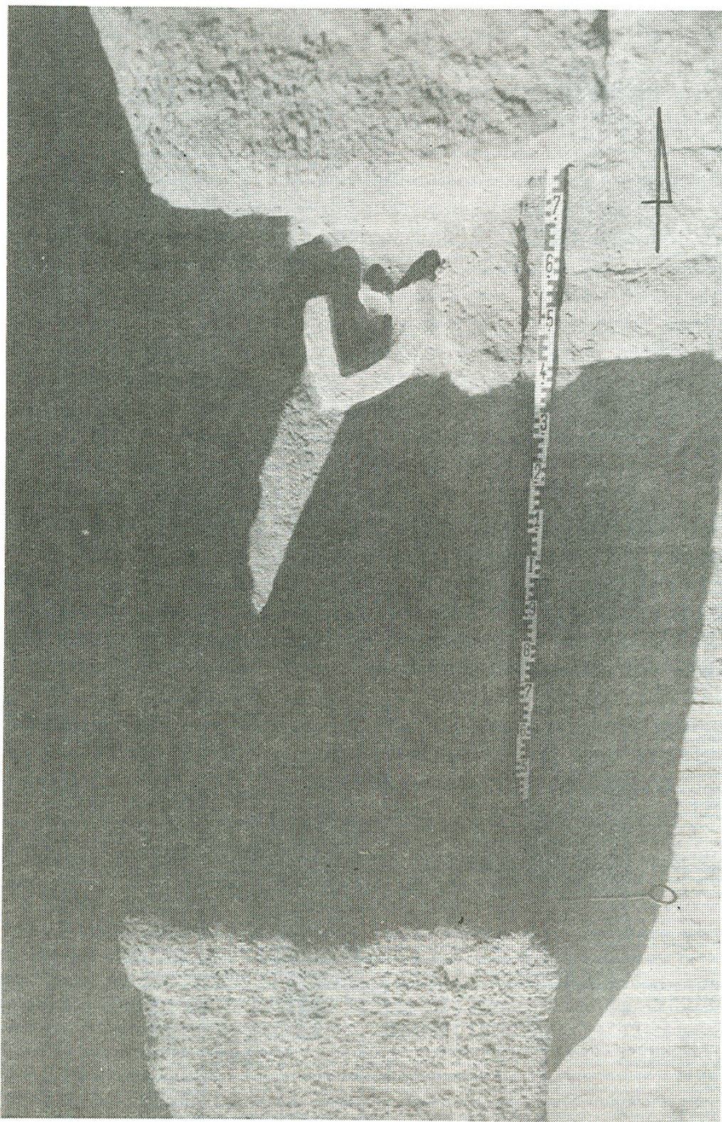
8. Qasr el-Sagha, Western Settlement 1988. Entrance leading to room No. 1 of unit C I (with the limestone "door-bed")
